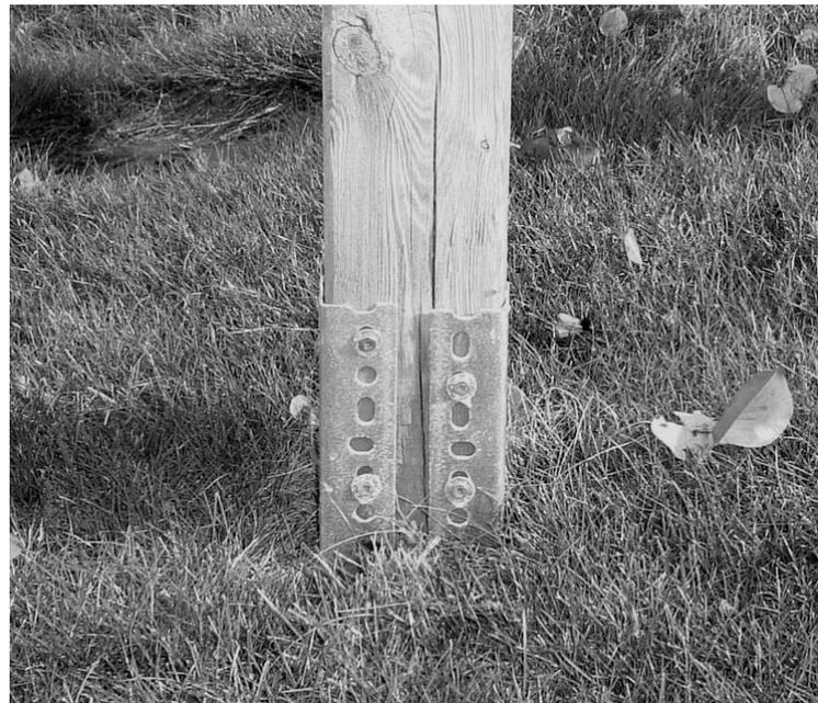
about \$10.00 and you can cut it into four pieces of 9". Leave about 5" above ground and 4" below ground and install one on each corner.  $\frac{3}{4}$ " x #10 Pan head screws should do the job of holding them on. Washers may be needed if the screw head is smaller than the hole. You can use cadmium plated screws but they will rust in a year or two. Try to get stainless steel screws and
