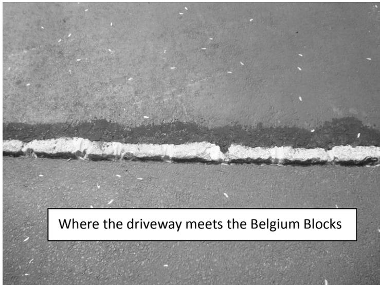
the caulking into any cracks or gaps and let it set up. You may have to repeat this because of shrinkage. If you have large areas or chunks missing use the patch material. Again, depending on the depth of the area you may have to repeat it if it shrinks. So do your repair and wait a day or two to see if you need
