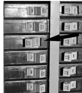
As fast as a circuit breaker stops the flow of electricity it will not open until it reaches the amperage rating of that particular breaker, for example, 15 or 20 amps. So if you were touching something in the house that
