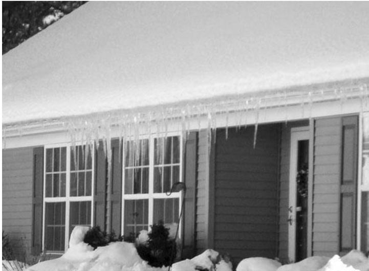
occurring, pull the insulation back away from the inside of the roof so air can reach it. If you have soffit vents, the same holds true. Insulation should not block the flow of cool air up from the soffit to the attic vents. Roofing experts do not usually recommend any kind of heating devices on the roof or gutters such as heat
